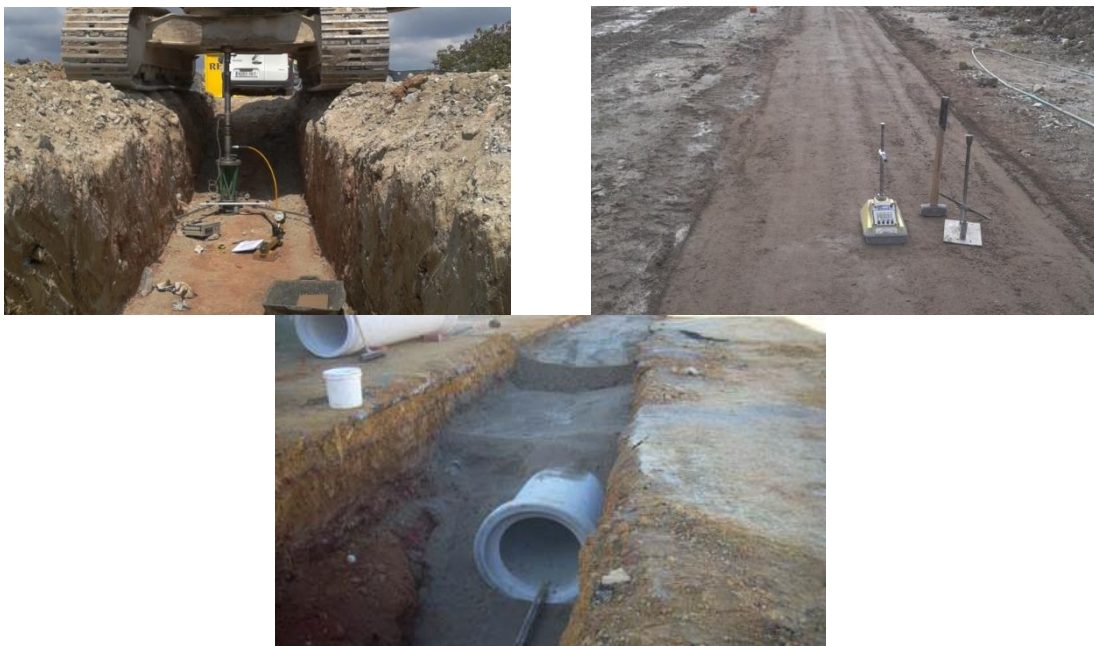
Image 1. Images from a restoration pipeline work. EMASESA
