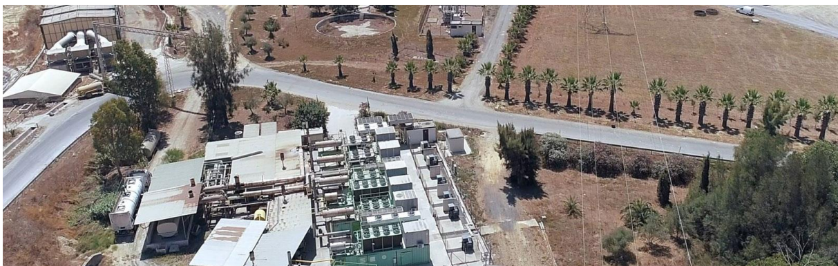
Image 3. View of Monte Marta Cónica Treatment Plant. Source: Aborgase web page: https://www.aborgase.com/
