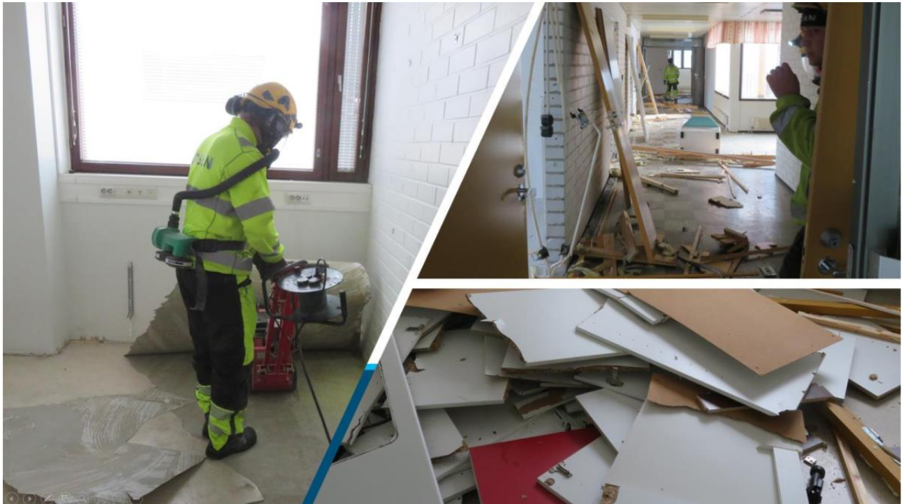
Conventional indoor demolition at Tuukkala Hospital
