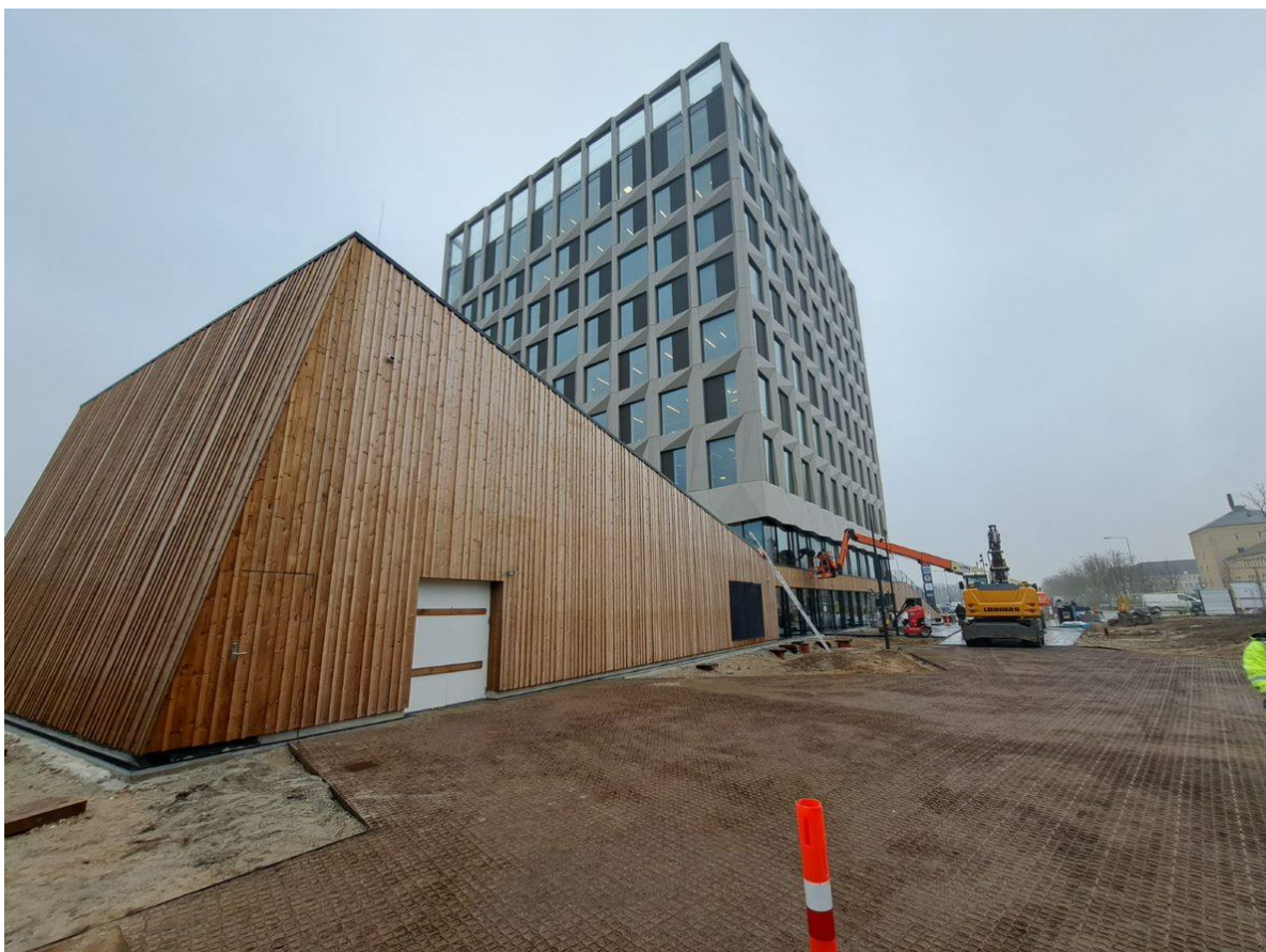
New city hall with outside wooden panels from offcuts (ground level and roof terrace)
