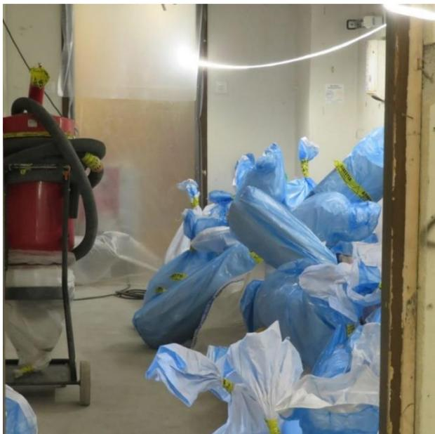
*Figure 9. Asbestos waste at Tuukkala site (photo Raimo Lilja)*
