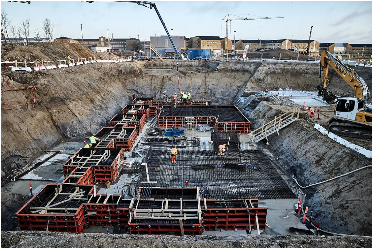
Figure 3: Making the foundation for Høje Taastrups new City Hall with recycled concrete (Photo: Unicon)
