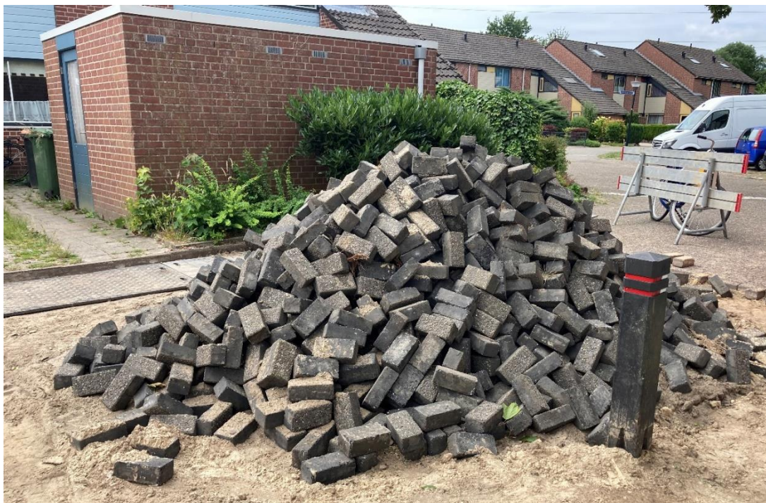
Figure 3.4. Used anthracite concrete pavers waiting on site to be reused in the parking spots.
