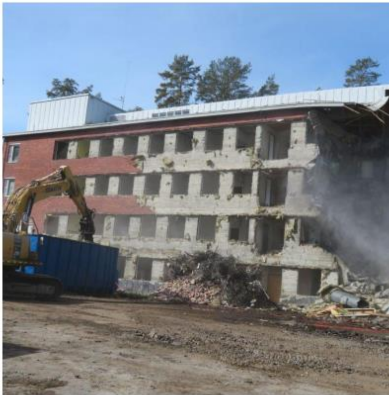
Figure 13 - Separate demolition of brick façade Mikkeli (photo Raimo Lilja)
