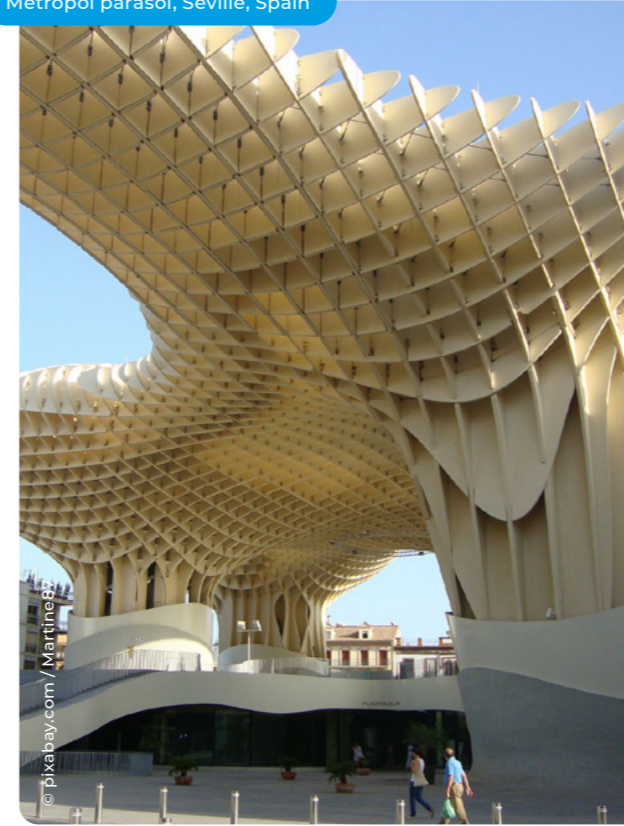
Metropol parasol, Seville, Spain
