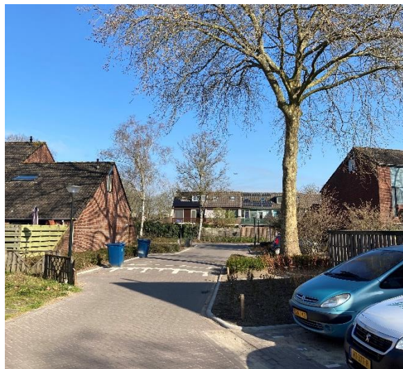
Figure 10: Parking space after renovating Griffiersveld where old concrete pavers were reused
