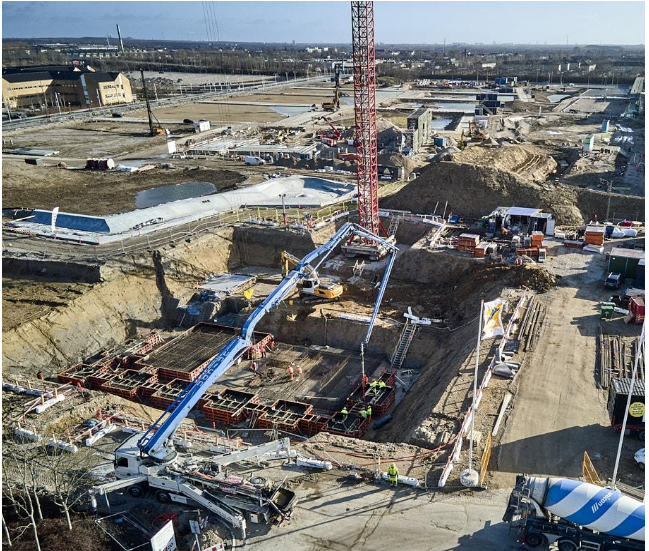
The construction site at the new City Hall I Høje-Taastrup from where excavated soil was transported 3 km away and reused under a football field (see next page)
