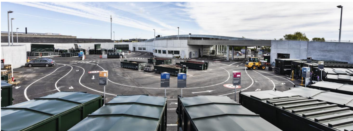
Fig. 11: South Harbour Recycling Centre in Copenhagen with a second-hand shop, test laboratory for teams of entrepreneurs to develop new products and circular business ideas and transform materials that would otherwise become waste into new products, and wholesale of large quantities of recycled materials to companies, individuals and organisations. Source: https://sydhavngenbrugscenter.kk.dk/
