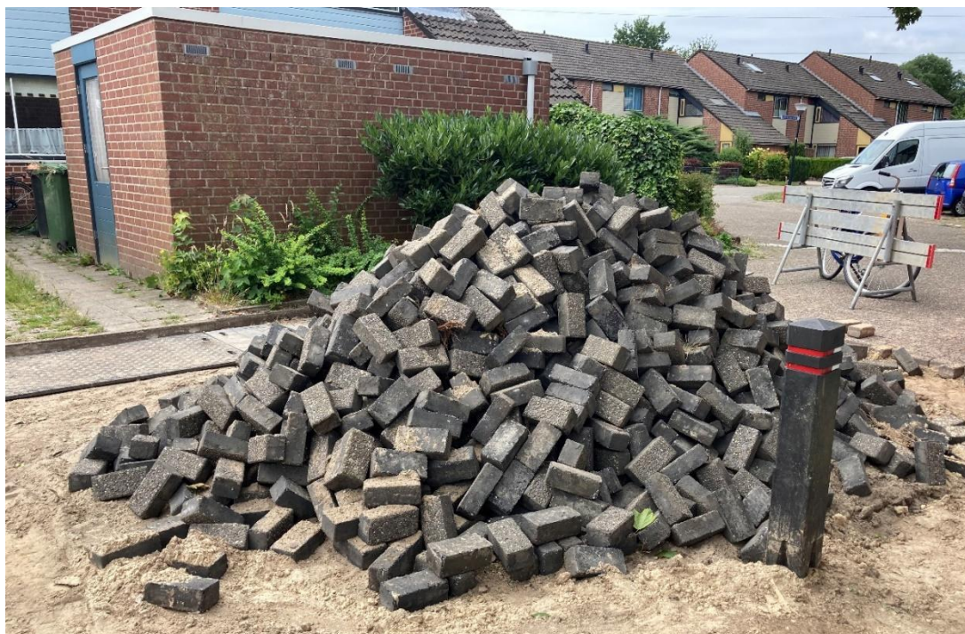
Figure 6. Used anthracite concrete pavers waiting on site to be reused in the parking spots.
