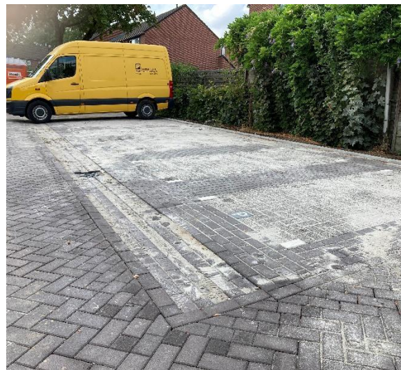
Figure 2. Parking space after renovating Griffiersveld where old concrete pavers were reused
