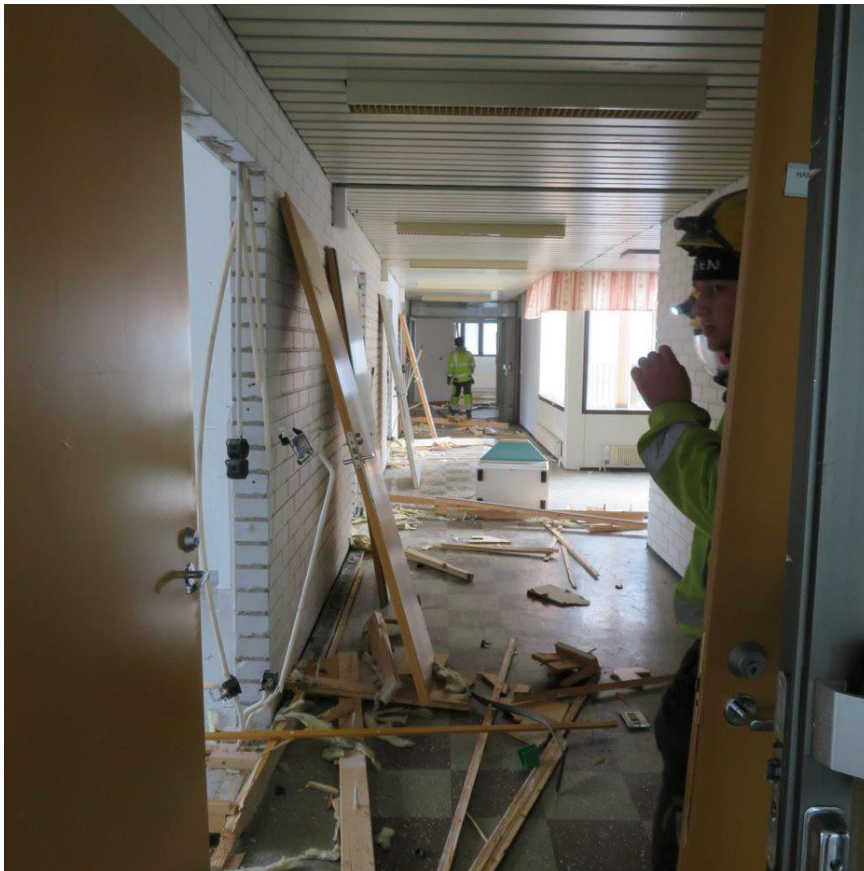
Figure 7. Indoor demolition (photo Raimo Lilja)
