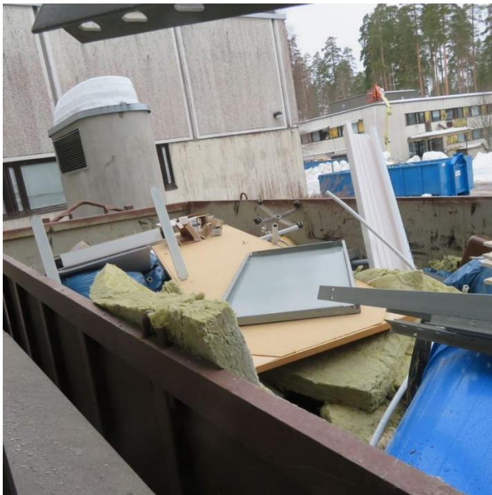
Figure 13. Example of mixed demolition waste (photo Raimo Lilja)
