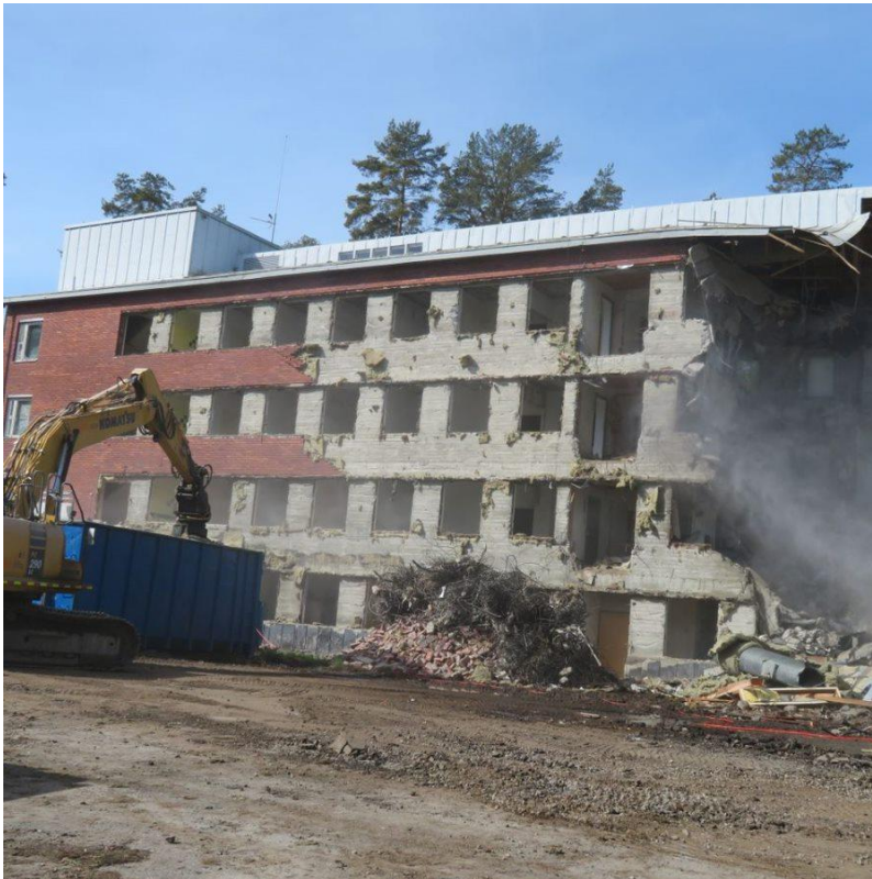
Figure 11. Separate demolition of brick facade (photo Raimo Lilja)
