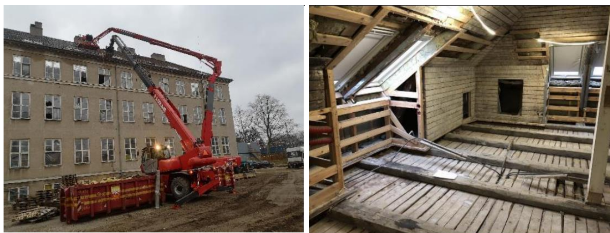
Figure 3 - Selective demolition of buildings, The Rockefeller-Centre, The National Hospital, Copenhagen 2018-2021. The photo left shows dismantling of roof tiles for reuse. The photo right shows interior locations after stripping of loose items, insulation etc. 15
