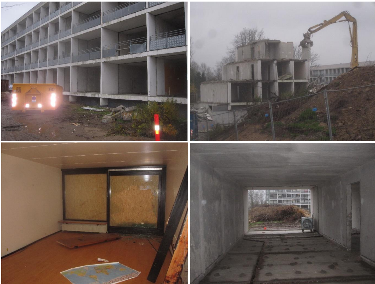
Figure 4 - Demolition of exposed residential building in Gellerupparken, Aarhus, 2015. The building is total stripped for interior materials and cleansed for contamination of PCB before demolition. After crushing on site all concrete materials are recycled and sold by the contractor.
