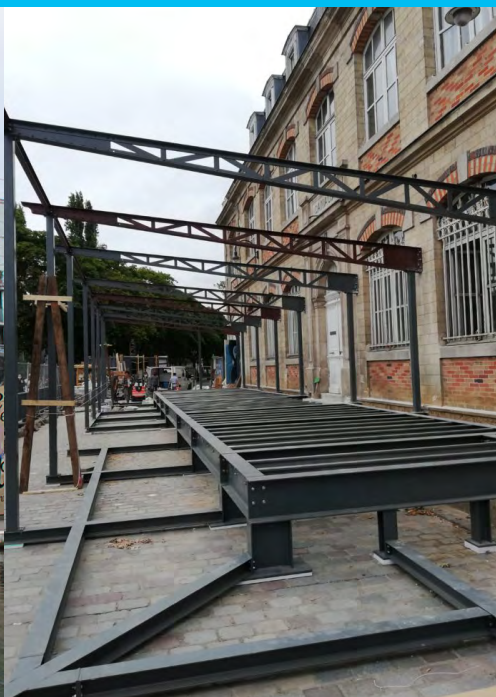
Les Canaux, a demonstration project for the City of Paris with reused materials - On the right, the reused metal structure of the terrace is provided from a demolished building closeby. © The City of Paris
