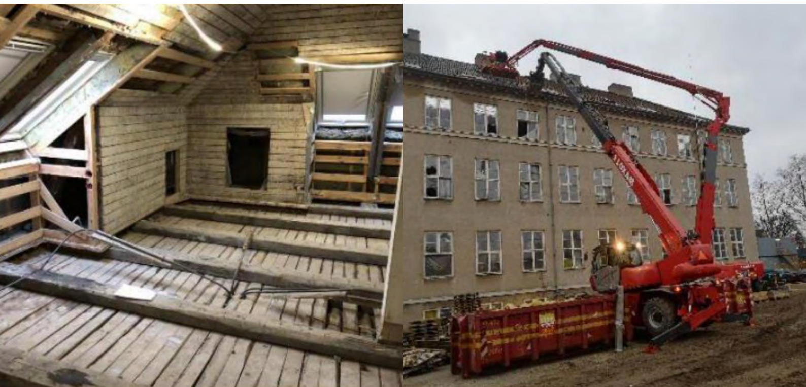
Selective demolition of buildings: The Rockefeller-Centre, The National Hospital, Copenhagen 2018-2021. The photo on the right shows dismantling of roof tiles for reuse. The photo on the left shows interior locations after stripping of loose items, insulation etc.
