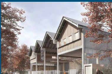
The urban factory has opened in September 2021 © Cycle Terre
