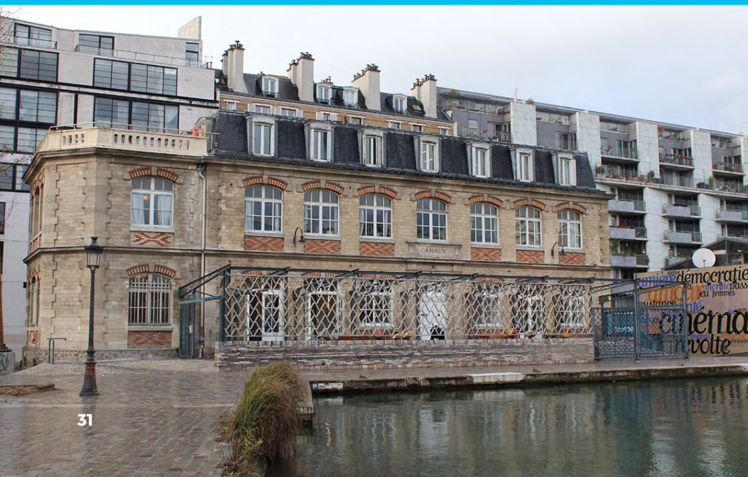
Les Canaux, a demonstration project for the City of Paris with reused materials - On the right, the reused metal structure of the terrace is provided from a demolished building closeby. © The City of Paris
