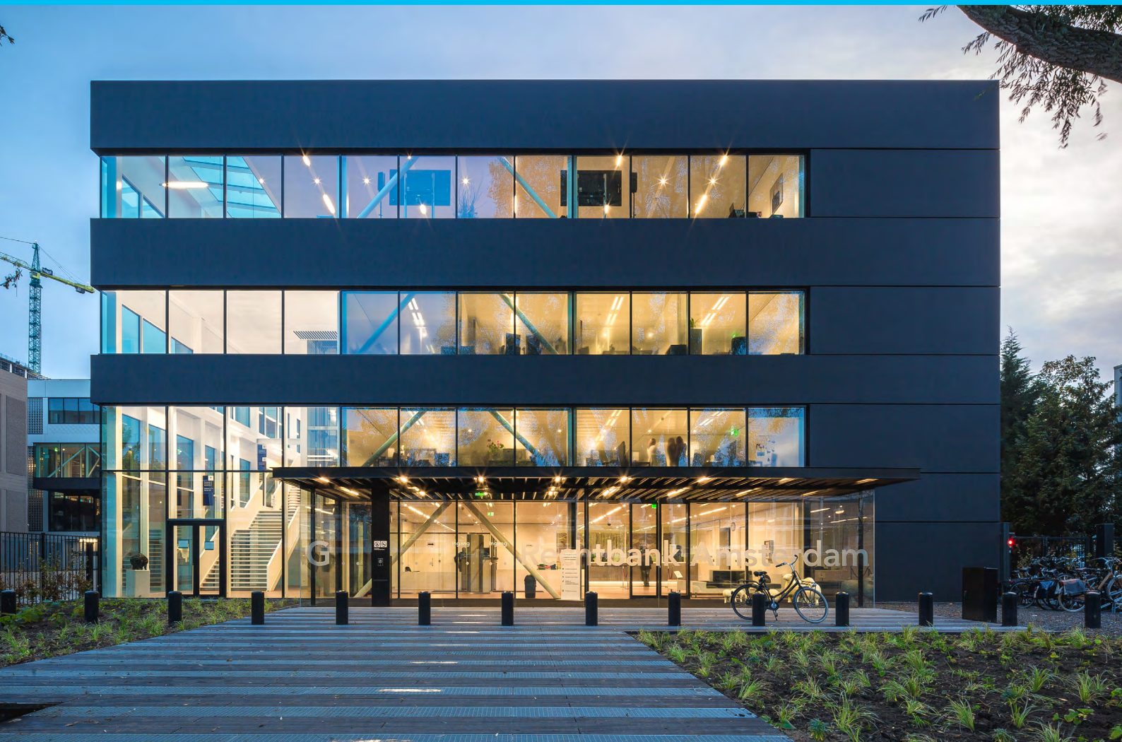
The temporary courthouse in Amsterdam. © cepezed | Léon van Woerkom
